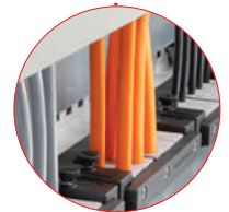
Straight cable routing into the cable duct
